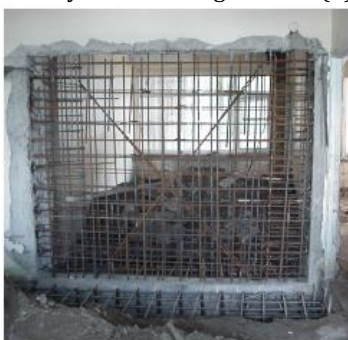
(a) additional shear wall
