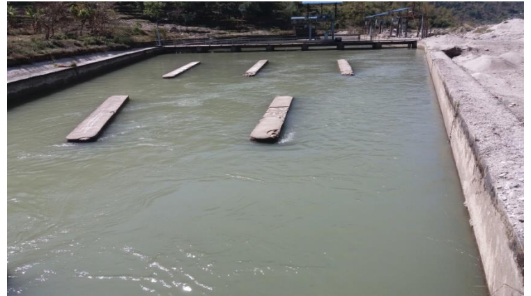
fig. Settling basin showing baffle wall
