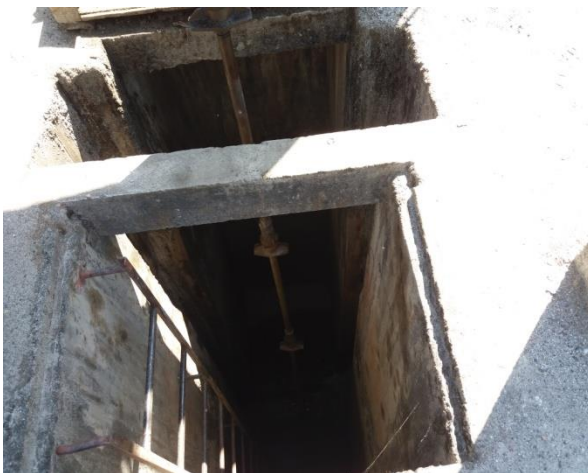
fig. flushing gate of settling basin
