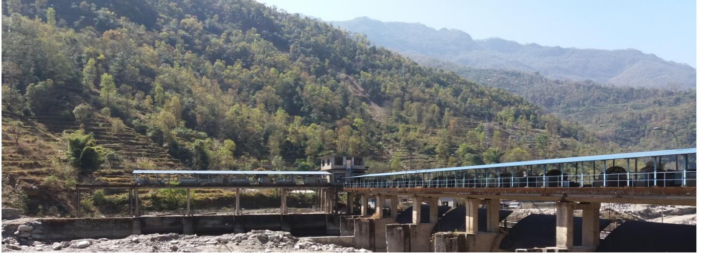
fig. Dam showing radial gates with hoist and intake
