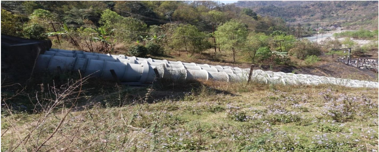
fig. three penstock pipes
