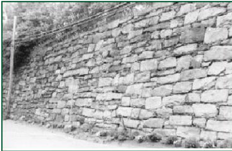
. Semi Gravity Retaining Wall
