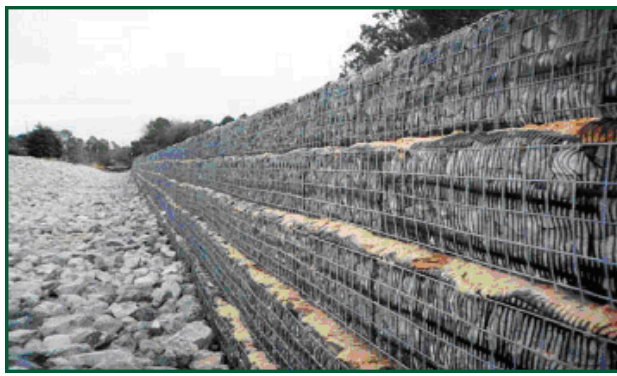
Fig. 6.9 (i) Gabion Wall
