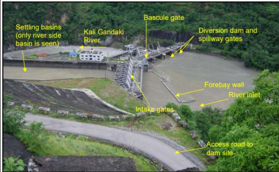
Existing headworks of Kali Gandaki A HPP during wet season operation
