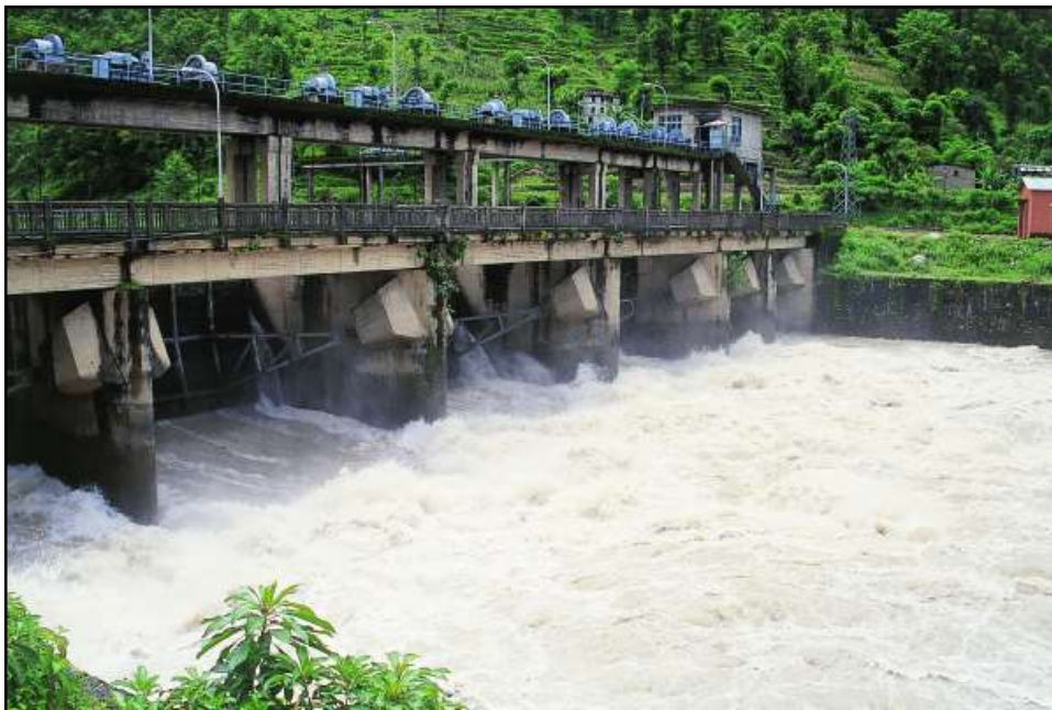
Sunkoshi barrage with hoisting room above
